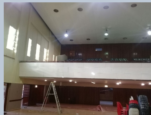
Repairs and renovations at Lenasia Civic Centre, Johannesburg
