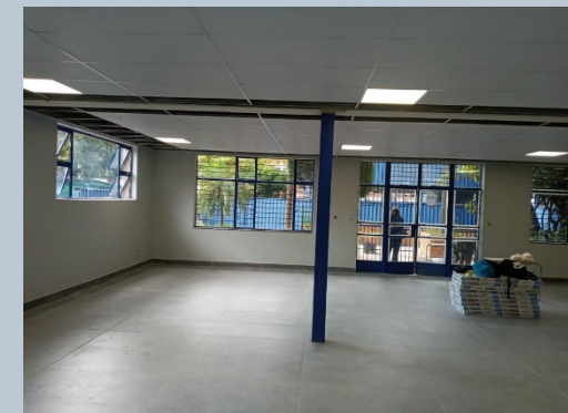
Refurbishment of Pretoria West Campus Canteen - Electrical
